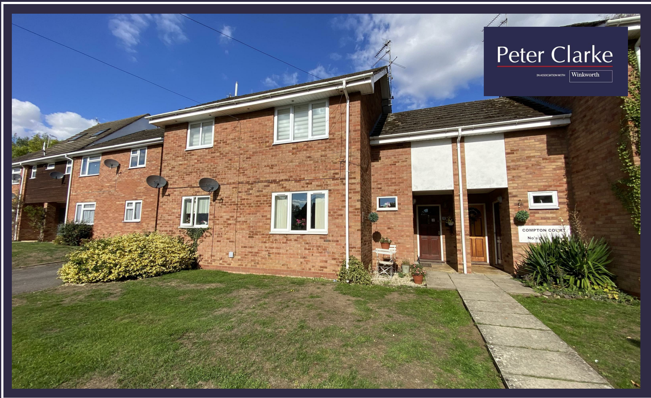
4 Compton Court Watery Lane, Shipston-on-Stour, CV36 4BE
